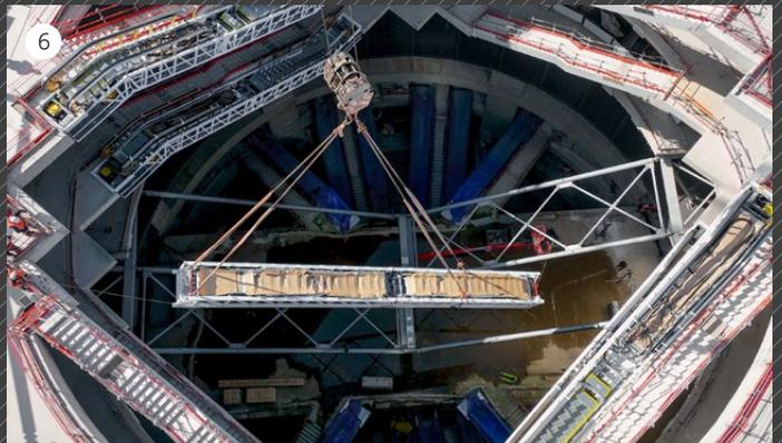
4 A crane lowers the escalators into the shaft, assisted by lifting straps.
