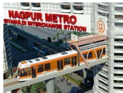
Nagpur Metro Rail project; Nagpur, India
