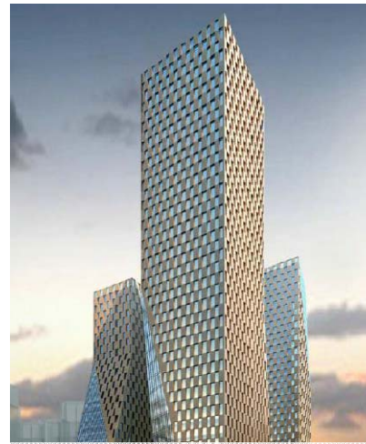
China Life building phase II; Hangzhou, China
