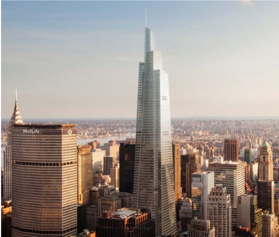
One Vanderbilt, 427m office and commercial tower; New York, USA
