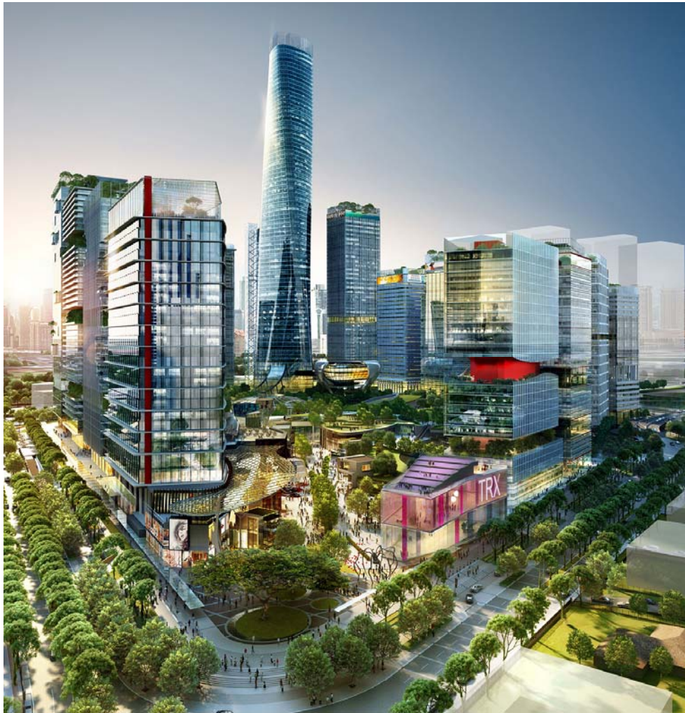
Signature Tower, office building; Kuala Lumpur, Malaysia 36 Schindler 7000 and 22 Schindler 5500 elevators, as well as 6 Schindler 9300AE escalators; PORT Technology.
