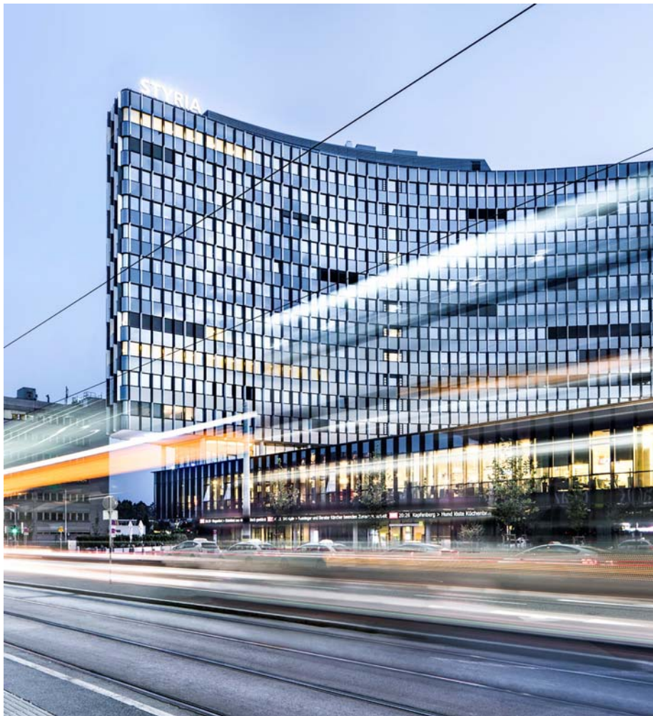
Styria Media Center, office building; Graz, Austria New installation of 7 Schindler 5500 elevators
