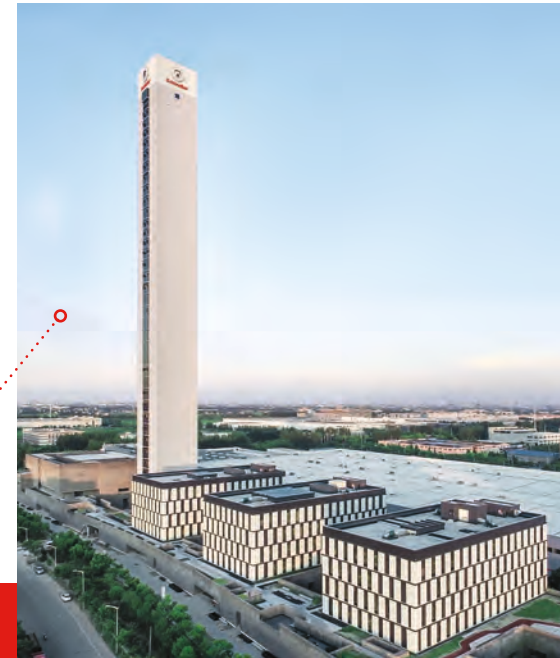
Schindler's Jiading campus in Shanghai, with factories, a 200m test tower, a R&D center, a training center, and the head office of Schindler China. It's been awarded a LEED Gold certification.
