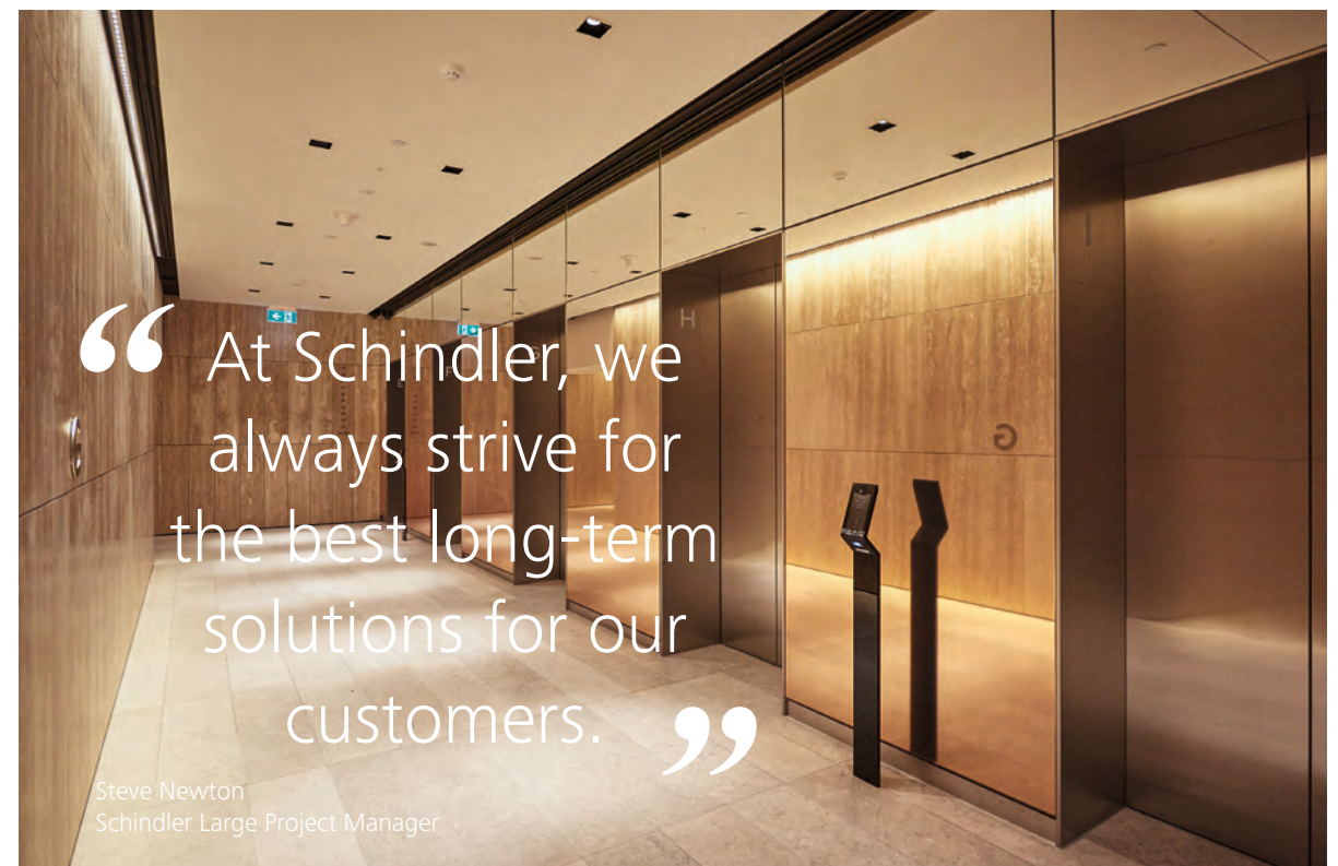
Landing hall of 80 Collins equipped with Schindler PORT terminals
