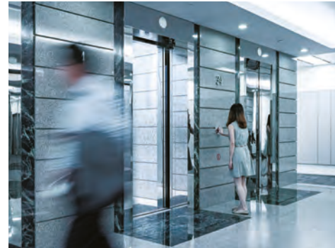
Landing hall of the plaza, equipped with Schindler PORT for a more efficient traffic management
