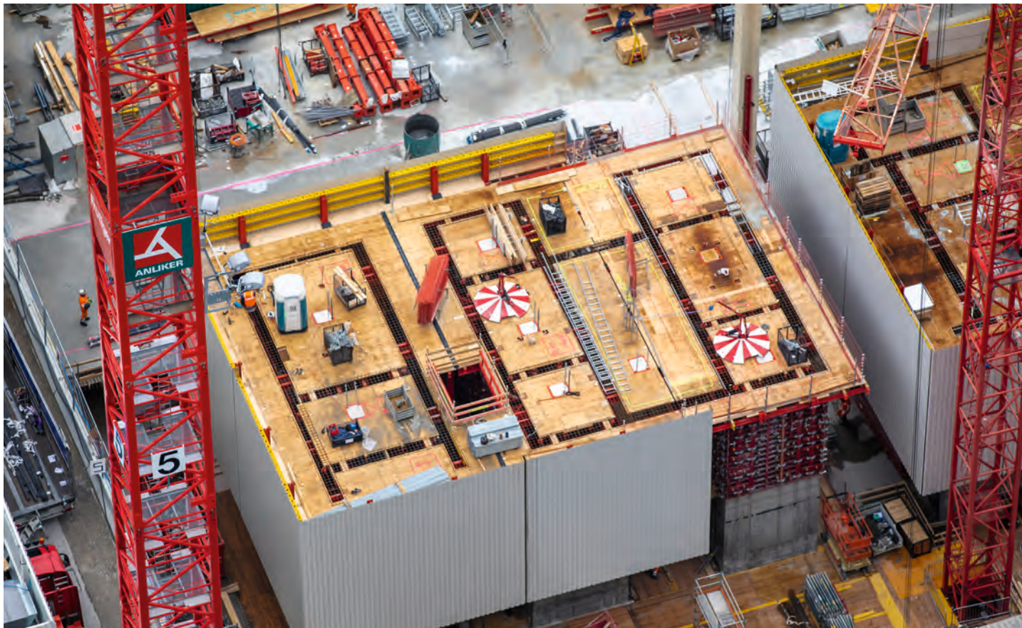
Construction site of pRED Center, Roche Site Basel, where Schindler CLIMB Lift was also applied
